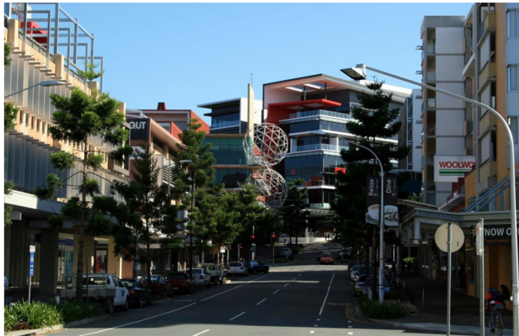
Fig. 7 Façade design and compact development
