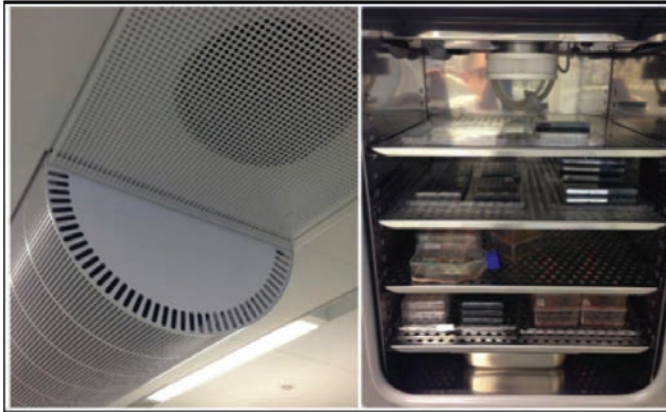
Figure 4. The ventilation system in the laboratories (left) created a low pressure, which sucked the stem cells out from the incubator as it was opened (the incubator is shown on the right).
