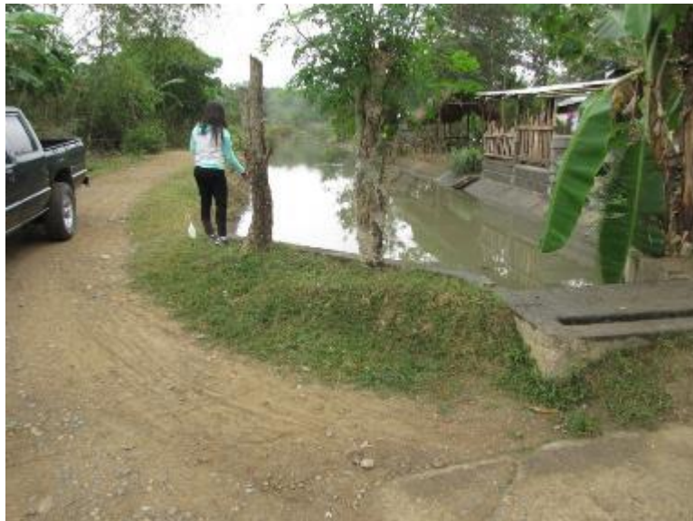
Photo 32. Main canal of Nungnung Dam (re-use dam), Div.4, MARIIS.
