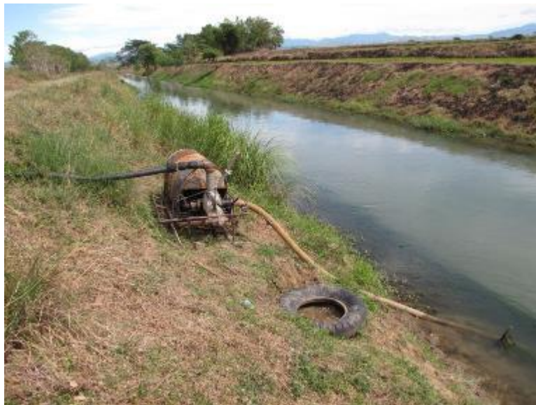
Photo 15. Illegal pumping unit along MC of LTRIS, Division 2, UPRIIS
