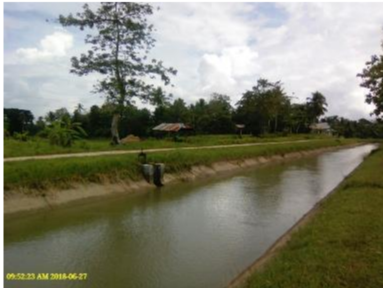
Photo 35. A direct turnout along MC of Malinao IS near Sta 0+00
