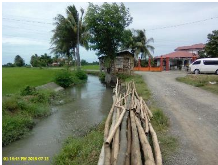
Photo 66. Section of the Main Canal, Suague RIS (midstream) with drainage intake (right side).
