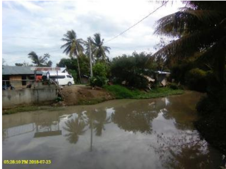
Photo 72. Illegal settlers along the drainage.
