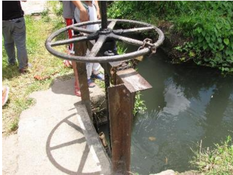
Photo 95. Gate in Cavite FLIS.
