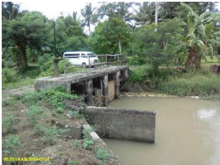
Photo 58. Check gate structure of Lateral B, Jalaur Proper RIS.
