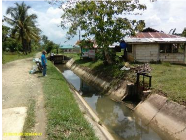
Photo 37. Section of Lateral D, Malinao IS in the downstream that are lined.
