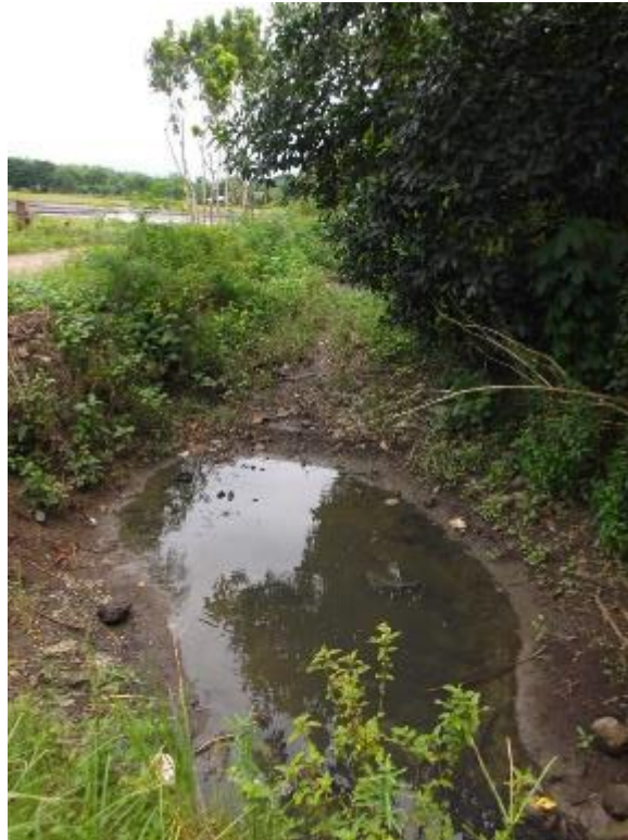
Photo 55. Downstream section of Lateral C, Jalaur Proper RIS.
