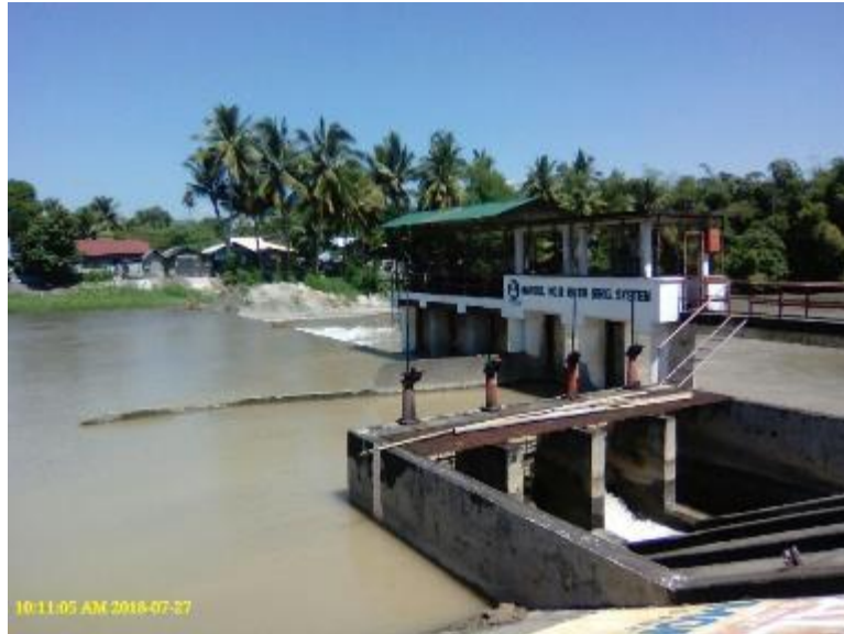
Photo 86. Diversion dam of the Marbel #2 RIS.
