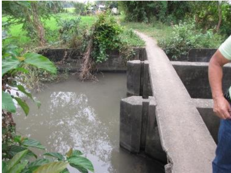
Photo 31. Check gate of Palomares Diversion Dam. One of the re-use dam in Div. 2, MARIIS.
