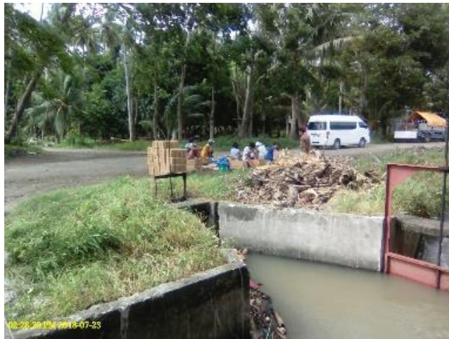
Photo 100. First (original) headgate of Lateral A of Padada RIS.
