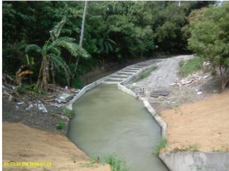
Photo 67. Newly lined headwater section of Padada RIS Main Canal.
