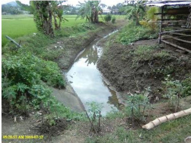
Photo 57. Section of Lateral B, Jalaur Proper RIS.
