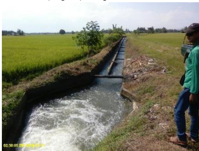
Photo 101. The "double" canal of Lateral F, Banga RIS.
