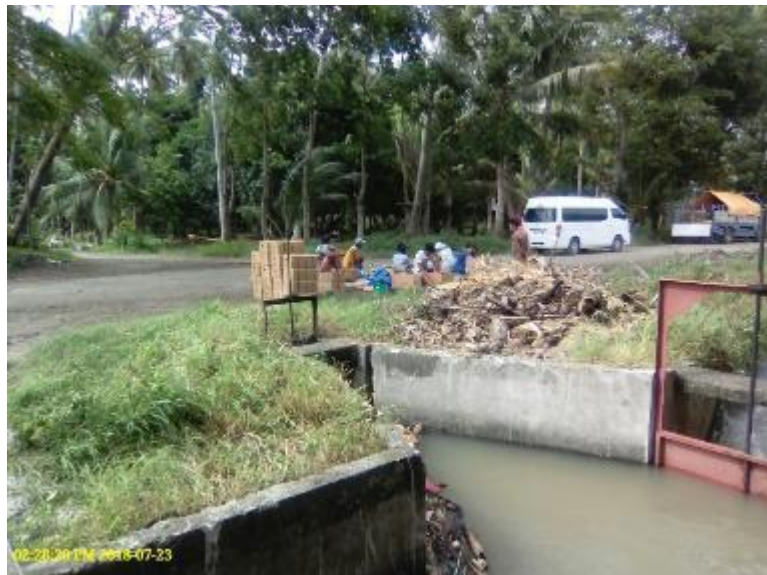
Photo 73. First intake gate of Lateral A.
