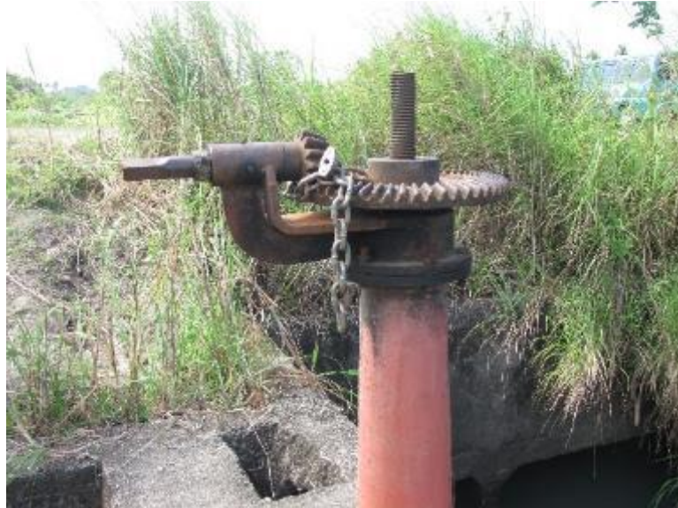
Photo 17. Check gate with padlocks in Libmanan-Cabusao PIS
