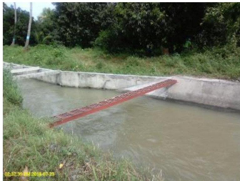
Photo 69. Bridge crossing over the Main canal of Padada RIS.
