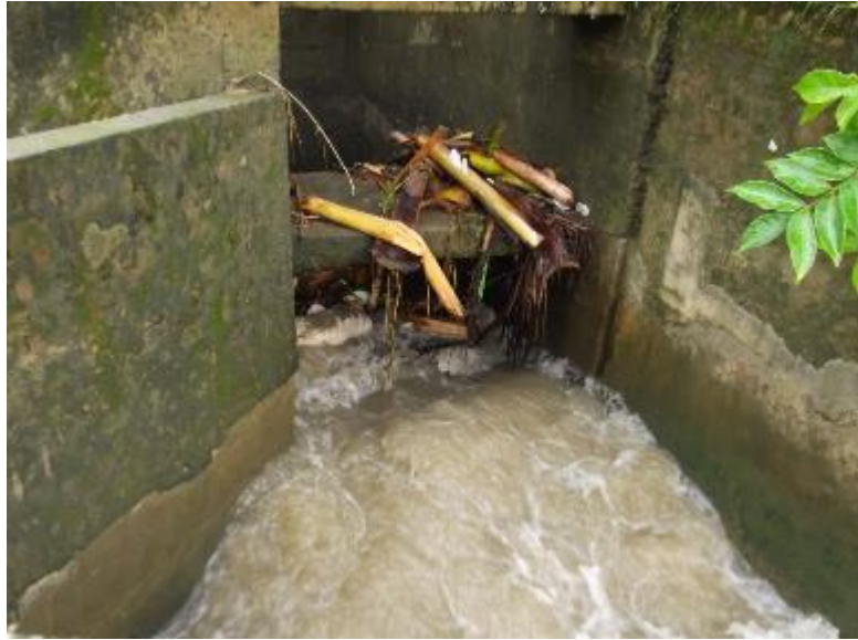
Photo 49. Clogged canal in Sibalom Tigbauan. (Take note of the dead swine together with the debris)
