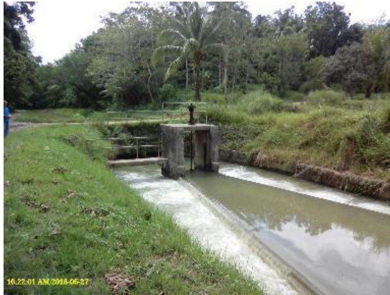
Photo 43. Duckbill weir near Lateral A, Malinao IS.
