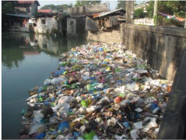
Photo 97. Section of Main Canal of Angat-Maasim RIS.
