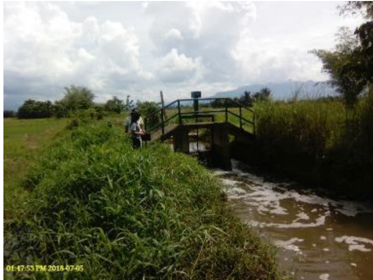
Photo 8. Belisong #1 dam (re-use dam) of Lower Binahaan RIS.
