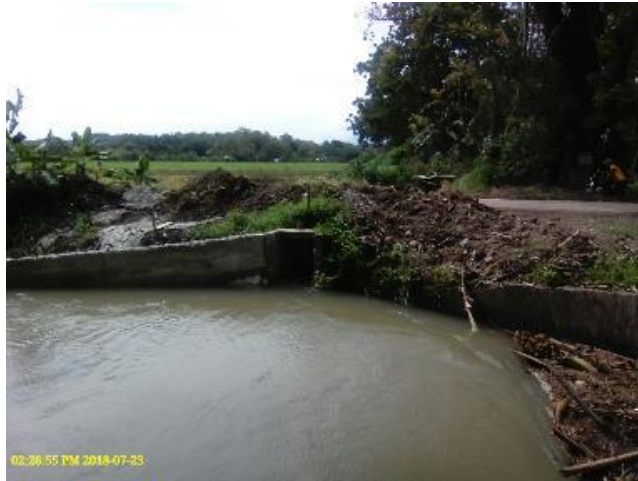
Photo 99. Second headgate of Lateral A of Padada RIS.
