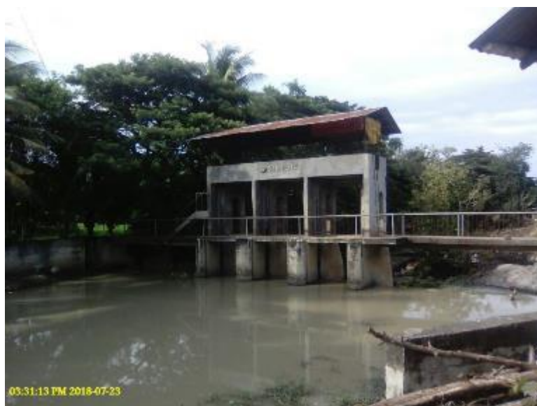
Photo 68. Parat dam along Sacub river (Intake dam for Padada RIS area).
