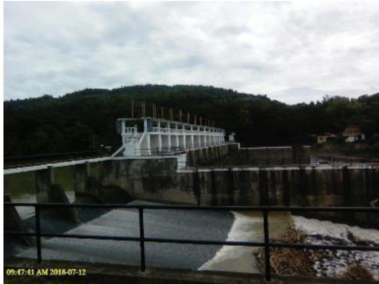
Photo 44. Diversion dam of Jalaur Proper and Jalaur Extension RIS.
