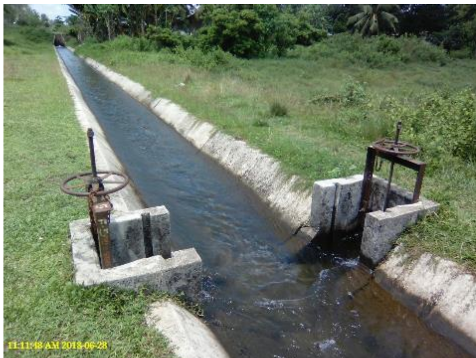
Photo 18. Section of Lateral C of Bayongan IS. Take note of the chains with padlock on the turning mechanism of the gates.
