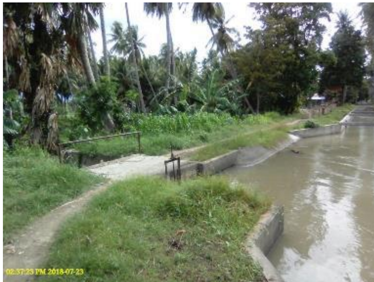
Photo 75. Silt ejector converted into supply gate opposite Lateral B headgate.
