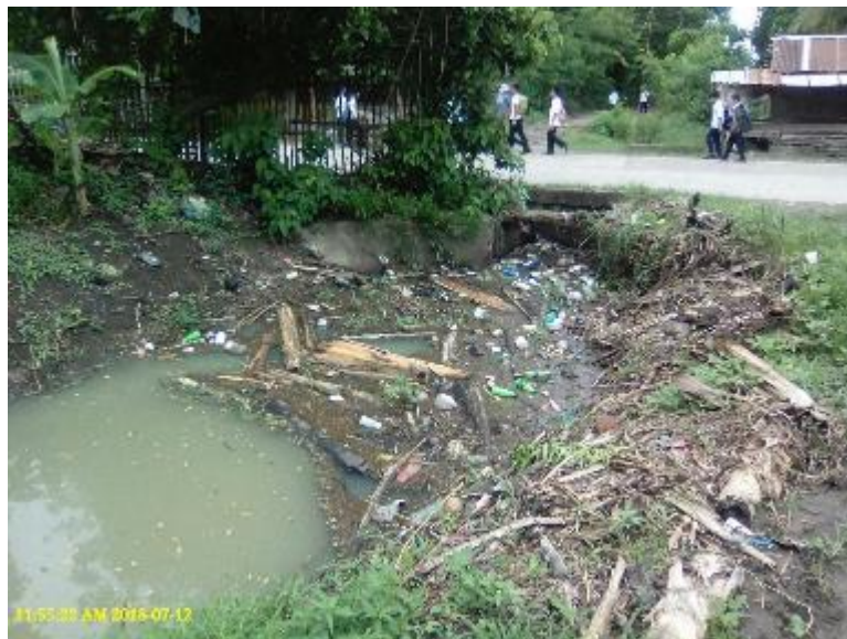
Photo 64. Downstream section of Lateral G, Jalaur Proper RIS.
