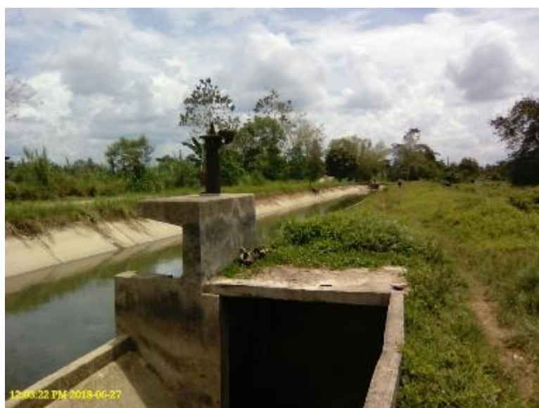
Photo 34. Gate of the spillway that supply water to Malinao IS to Bayongan reservoir
