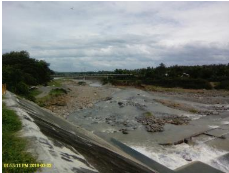
Photo 70. Problem at the dam site due to over quarrying near the downstream section of Padada RIS dam.
