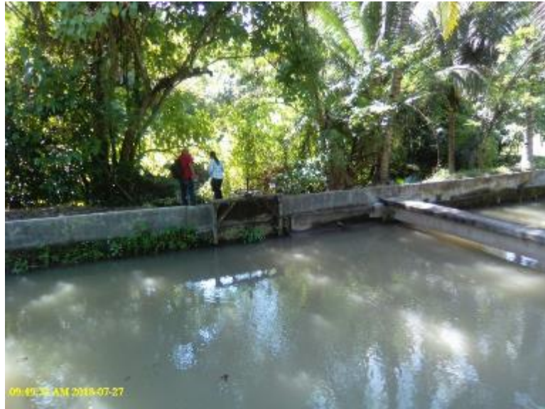
Photo 88. Control gate of one of the wasteways of Marbel #1 RIS.
