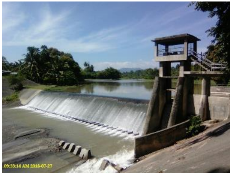
Photo 82. Diversion dam of Marbel #1 RIS.
