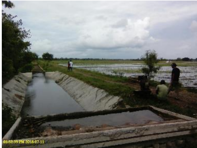
Photo 53. Lined section of Lateral F, Jalaur Extension RIS.
