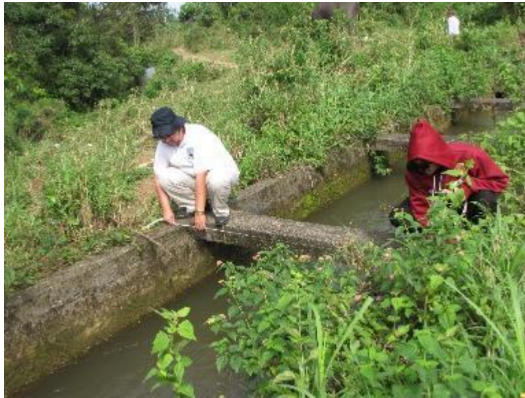
Photo 90. Section of Main Canal of Visitacion NIS
