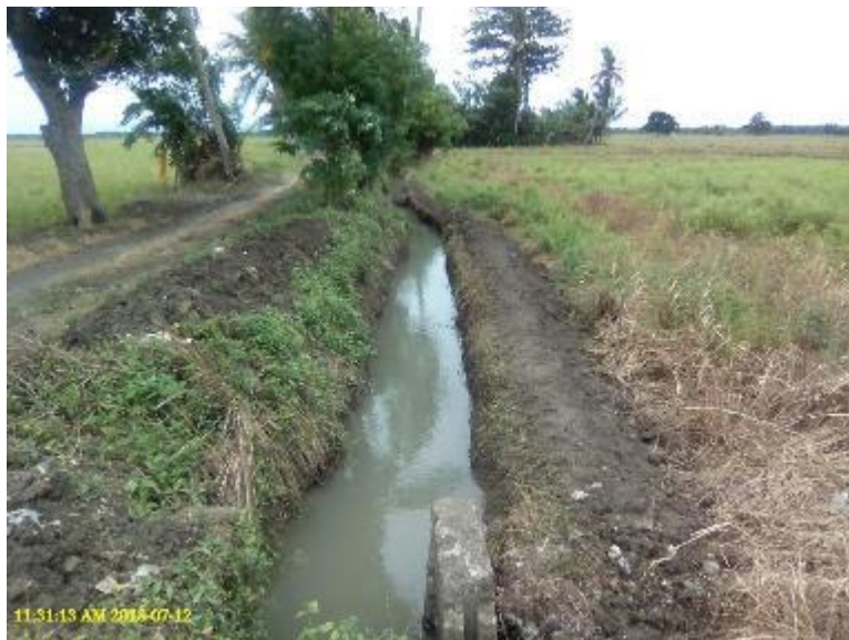
Photo 62. Newly-cleaned main farm ditch in Jalaur Proper RIS.
