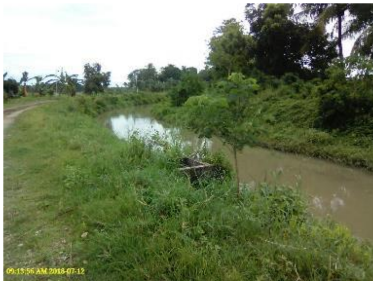
Photo 56. Direct turnout along Main Canal, Jalaur Proper RIS.
