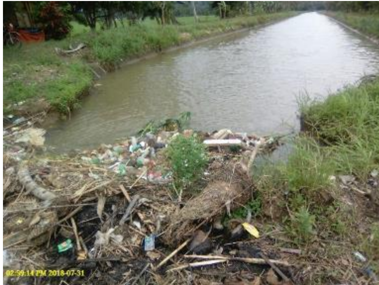
Photo 14. Section of South Main Canal of Pulangui RIS with floating debris trapped in a headgate.
