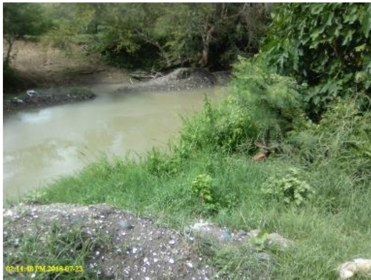
Photo 2. Silted Main Canal of Padada RIS where presence of shellfish is evident.
