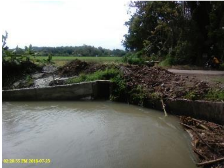
Photo 74. Second intake gate of Lateral A.
