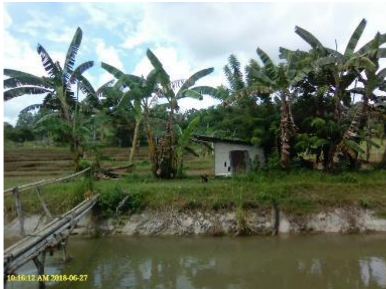
Photo 36. A pumphouse along MC in the upstream section of Malinao IS.
