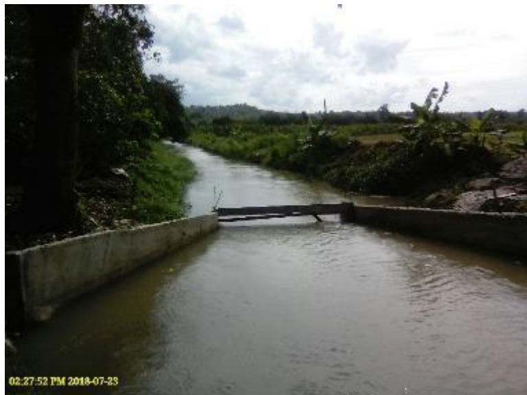
Photo 94. Unfinished construction of Main canal of Padada RIS near Lateral A.
