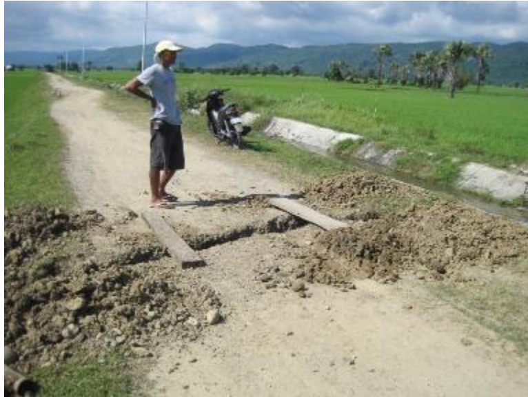
Photo 16. Illegal turn out along lateral of Caguray RIS (Photo courtesy of Engr. Wilson Lopez)
