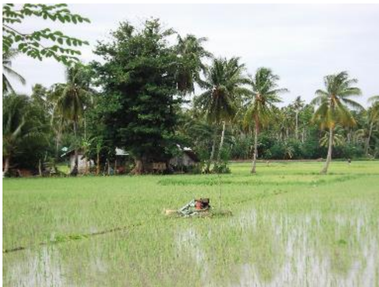
Photo 12. A pumpset installed in the service area of Padada RIS.
