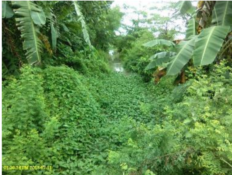
Photo 51. Vegetations that clogged the end check and drainage out let of Jalaar Extension RIS.
