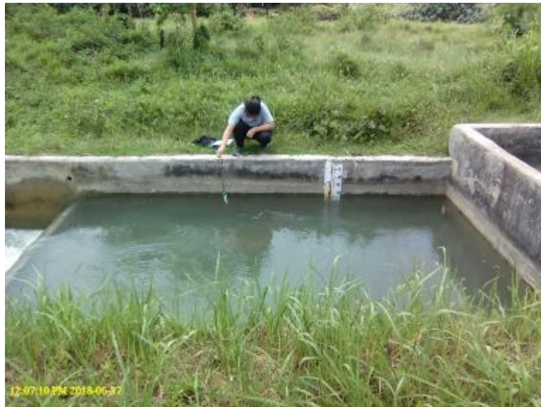
Photo 38. Staff gage installed in the downstream section of Malinao IS MC.
