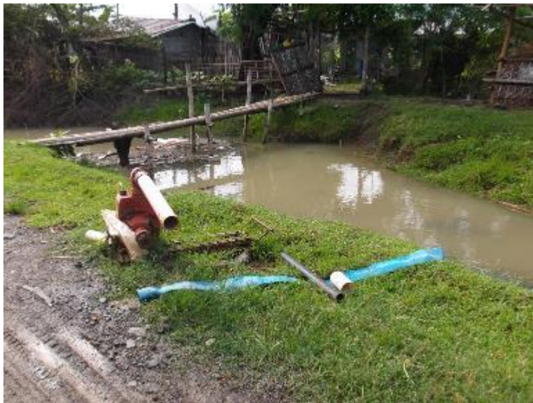
Photo 10. A pumpset installed along Main Canal, Sibalom-Tigbauan RIS (downstream section).
