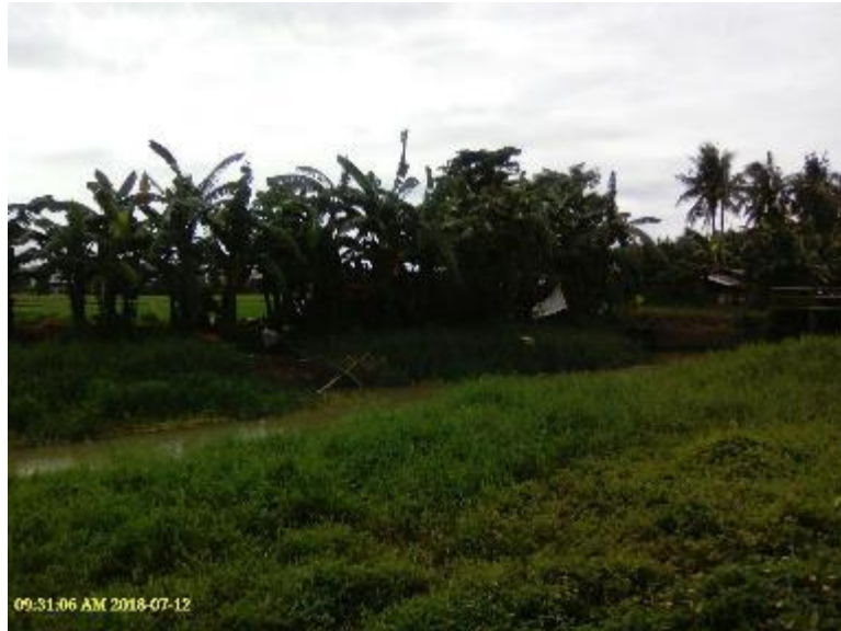
Photo 59. A pumpset along Main Canal, Jalaur Proper RIS. Take note of the width of the canal and vegetations along.
