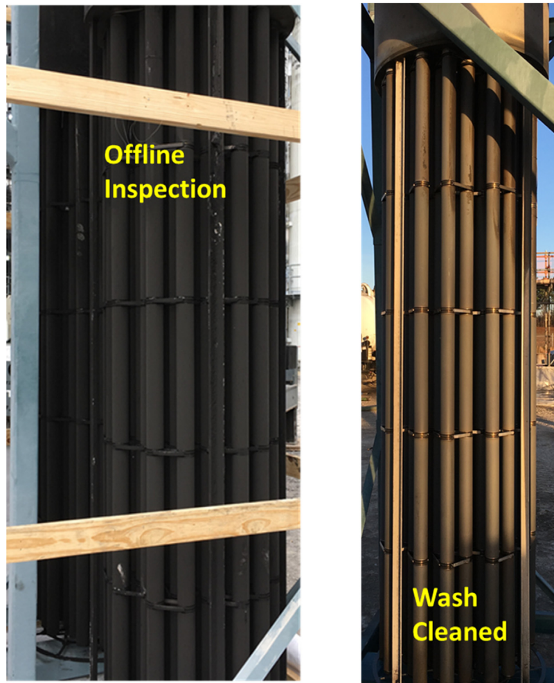
Fig. 11. Filter elements after an on-coal operation.
