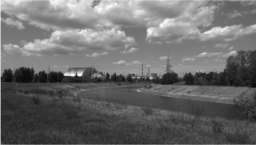
Figure 2.1 Panorama of the Nuclear Power Plant.
