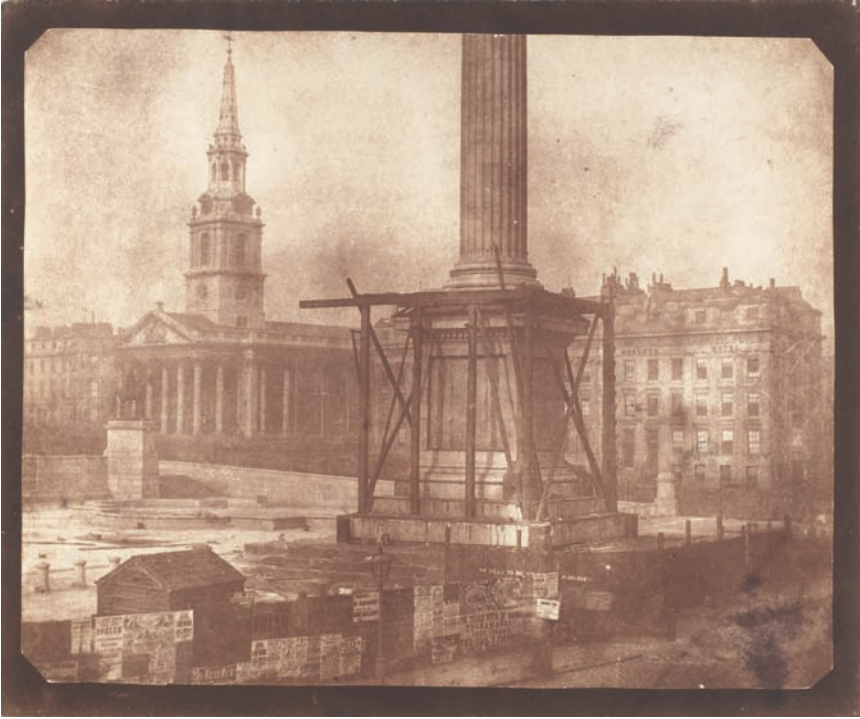
Figure 3.4 William Henry Fox Talbot, Nelson's Column under construction, Trafalgar Square, first week of April 1844.
