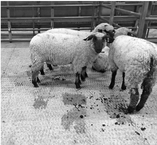
Figure 12.8 A good non-slip flooring surface that can be used for sheep or pigs. It is created by stamping the pattern of expanded metal mesh into the wet concrete. For cattle, a slightly deeper pattern is recommended (photo credit: Temple Grandin).
