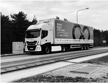
Image 5.1 Smart road system in Gotland, Sweden. Source: Smartroad Gotland.
