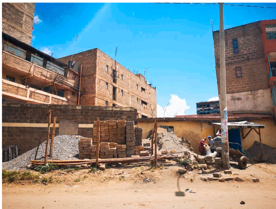
Fig. 7. Building materials sale along Mathare Road. For bulky materials are stone and gravel, retailers rely on the available street surface or open plots, whereas available. The stone blocks here stocked for sale are second-hand materials, collected from a nearby demolition site, and are a rarity within the local market.
