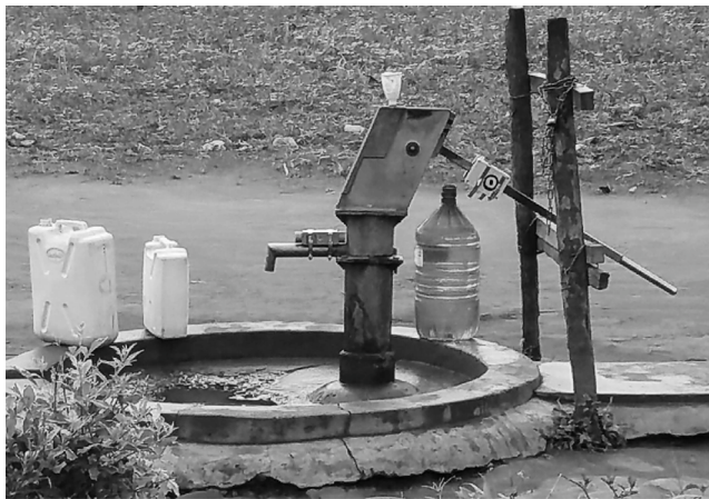
Fig. 1. India Mark II hand pump. Source: photo by the authors.
