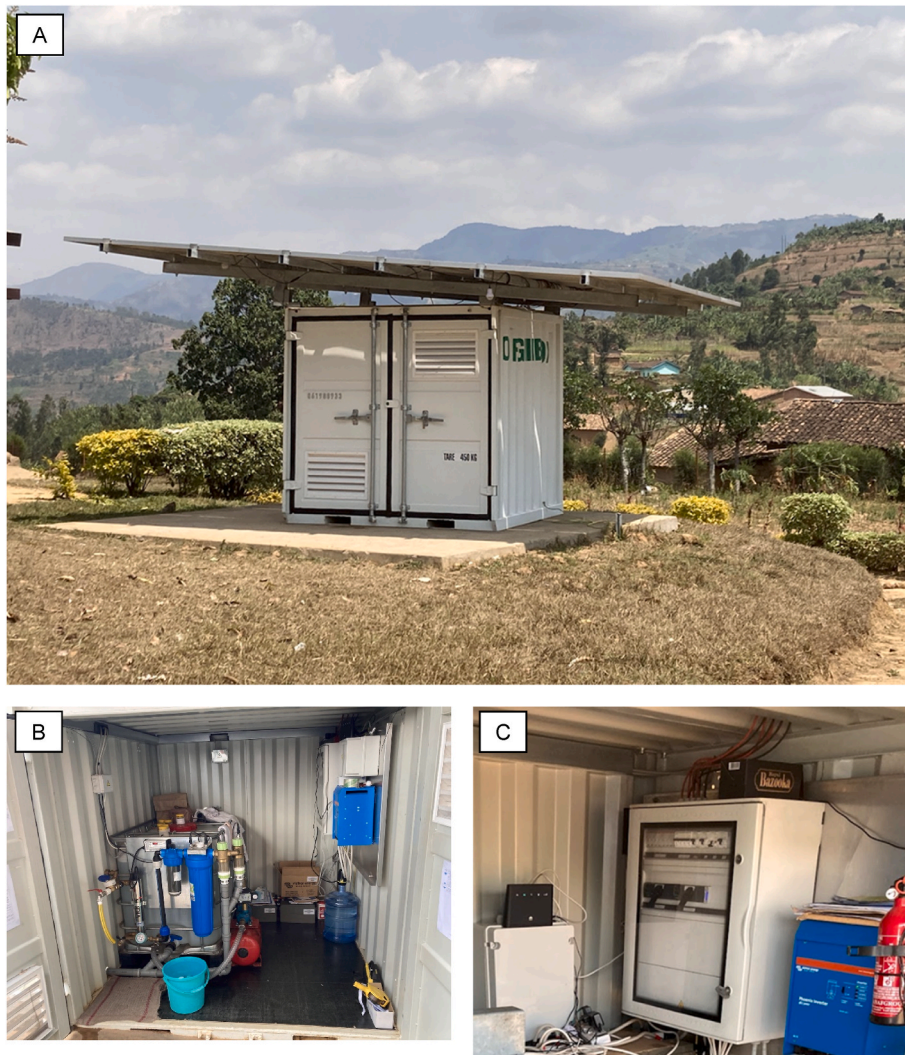
Fig. 5. (A) A deployed Box. (B) View of water module inside Box. (C) View of internal power module elements. Photos by S. Miles.
