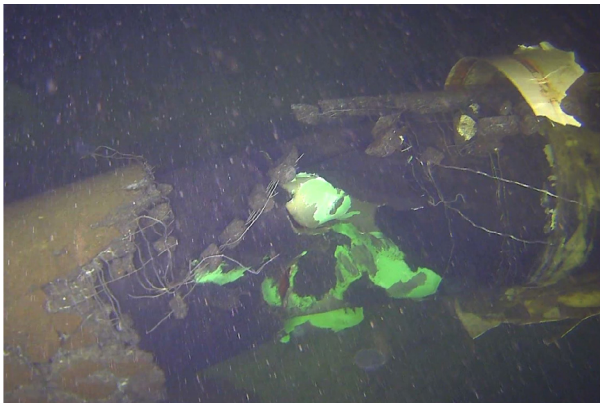
Figure 4. The damaged Balticconnector gas pipeline, October 2023
