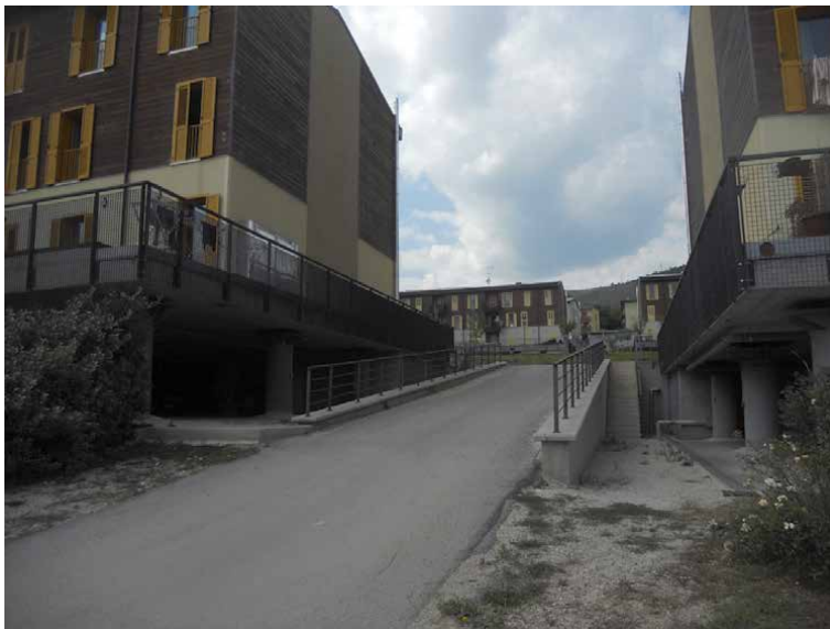
Figure 24. Temporary residences built around L'Aquila under the government of Silvio Berlusconi. Note the ground insulators (photo S. Gizzi, 2013).
