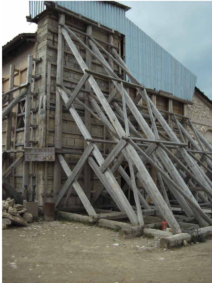
Figure 17. Shoring of the church of Onna (photo S. Gizzi, 2011).
