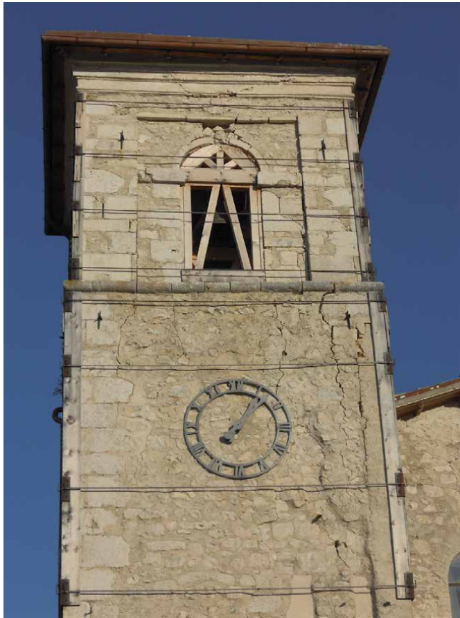
Figure 15. Provisional works in San Martino d'Ocre (Photo S. Gizzi, 2011).
