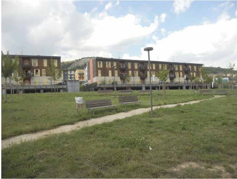
Figure 23. Temporary residences built around L'Aquila under the government of Silvio Berlusconi (photo S. Gizzi, 2013).
