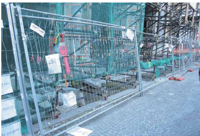
Figure 27. L'Aquila, the keys to the houses declared uninhabitable hung by the inhabitants, as a sign of protest, along Corso Vittorio Emanuele II (photo S. Gizzi, 2010).
