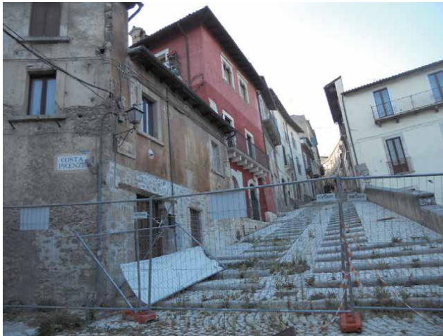
Figure 25. L'Aquila, the "red zone" of via Costa Masciarelli, in the historic center (photo S. Gizzi, 2011).
