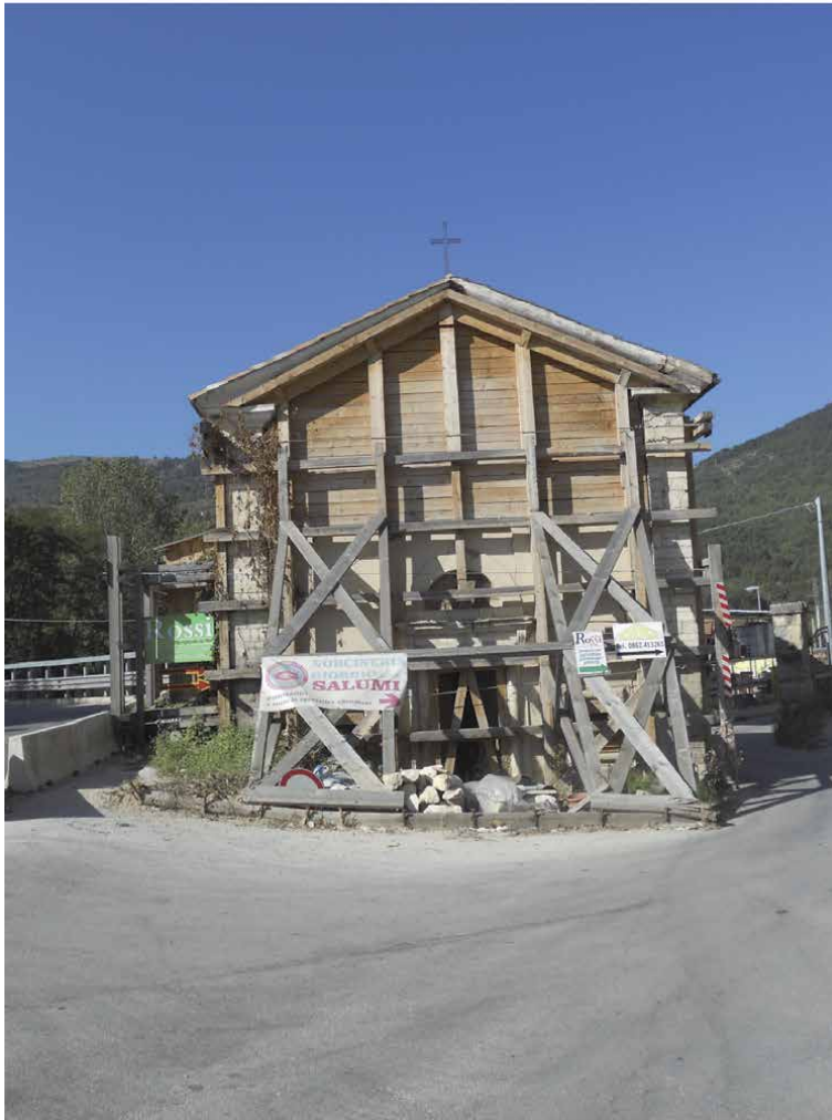
Figure 12. “Works in wood provisional in a small church outside the city walls” (photo S. Gizzi, 2011).
