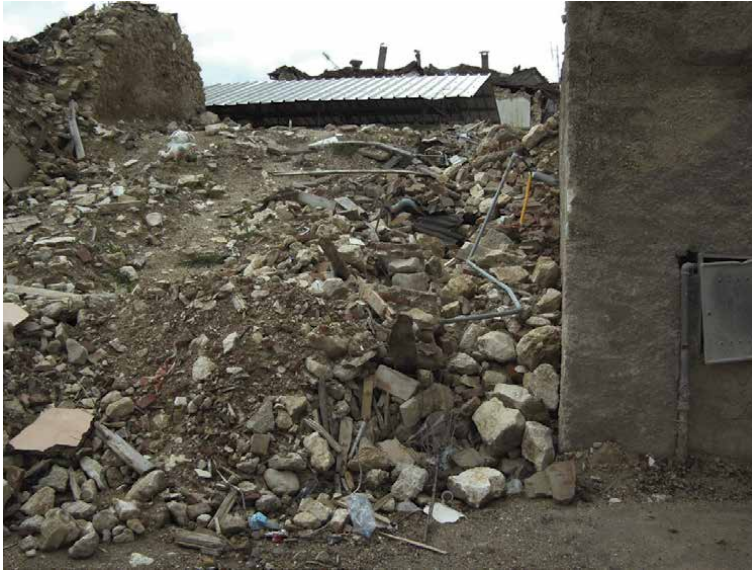
Figure 33. Onna, near L'Aquila. Collapses and rubble (photo M. M. Segarra Lagunes, 2011).
