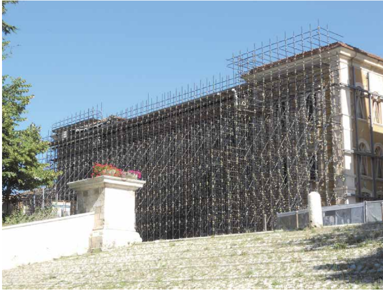
Figure 9. Dense scaffoldings near the basilica of San Bernardino (photo S. Gizzi, 2011).
