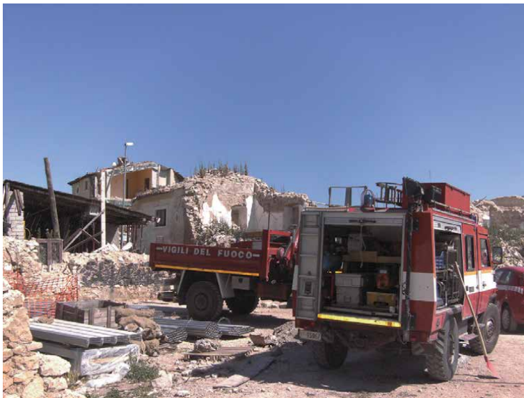
Figure 36. Fire brigade in Onna, after the collapses (photo S. Gizzi, 2010).
