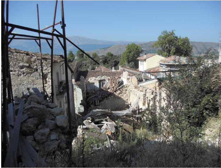
Figure 35. Collapses in Paganica, a hamlet of L'Aquila (photo S. Gizzi, 2011).
