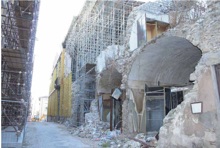
Figure 31. L'Aquila, collapses and props along the axis of Via Roma (photo S. Gizzi, 2010).
