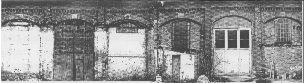
Illustration 18: Former Lokschuppen (Locomotion Barn), South Side, state in 1996
