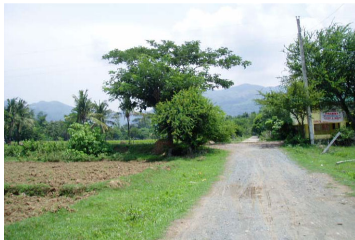
Figure 3.1 Typical Rural Road in the Philippines
