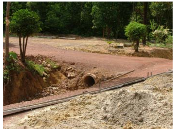
Erosion related to road building
