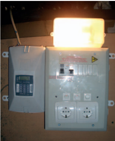
Some Households – most of them in Matola J – have also been equipped with a ready-board, a so-called „Quadrolec“.
