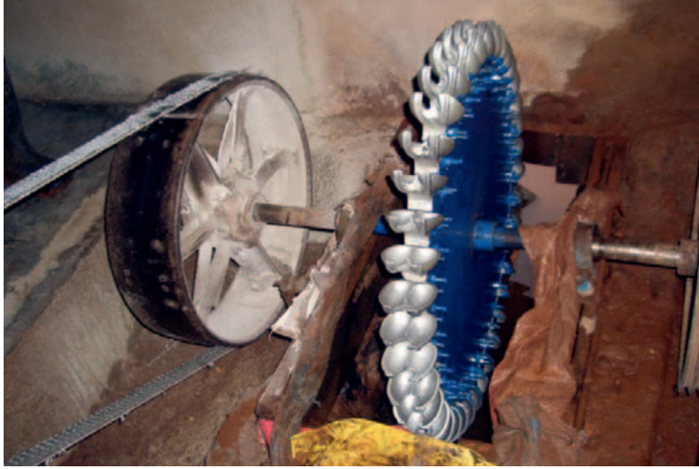
A second maize mill, already after its rehabilitation.
