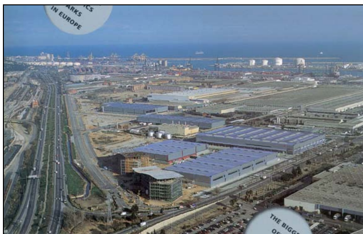
Figure 1: Parc Logistic under construction Source: El Consorci de la Zona Franca, 2002
