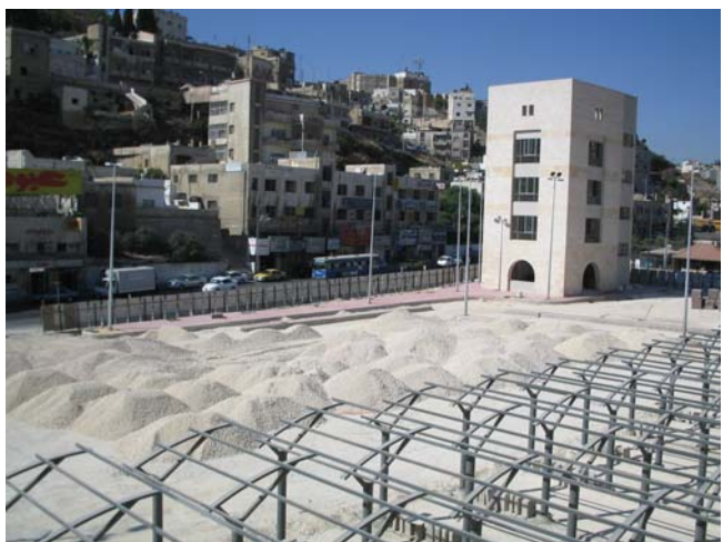
Picture 3. Raghadan Bus Terminal construction site
